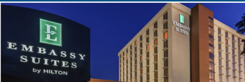
Embassy Suites Dallas Dallas, Texas Renovation
